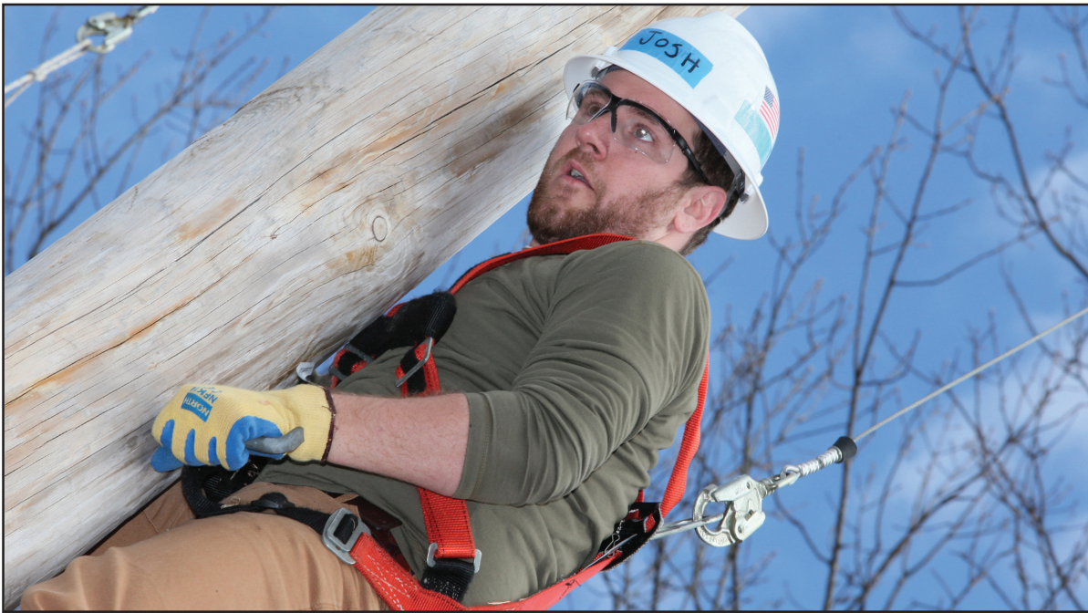
CCRI Energy Utility Technology Certificate student Josh Pomplun of Providence climbs a pole at the National Grid training facility in Millbury, Mass. Students spend 64 hours learning to service utility wires at the facility during their second semester.
